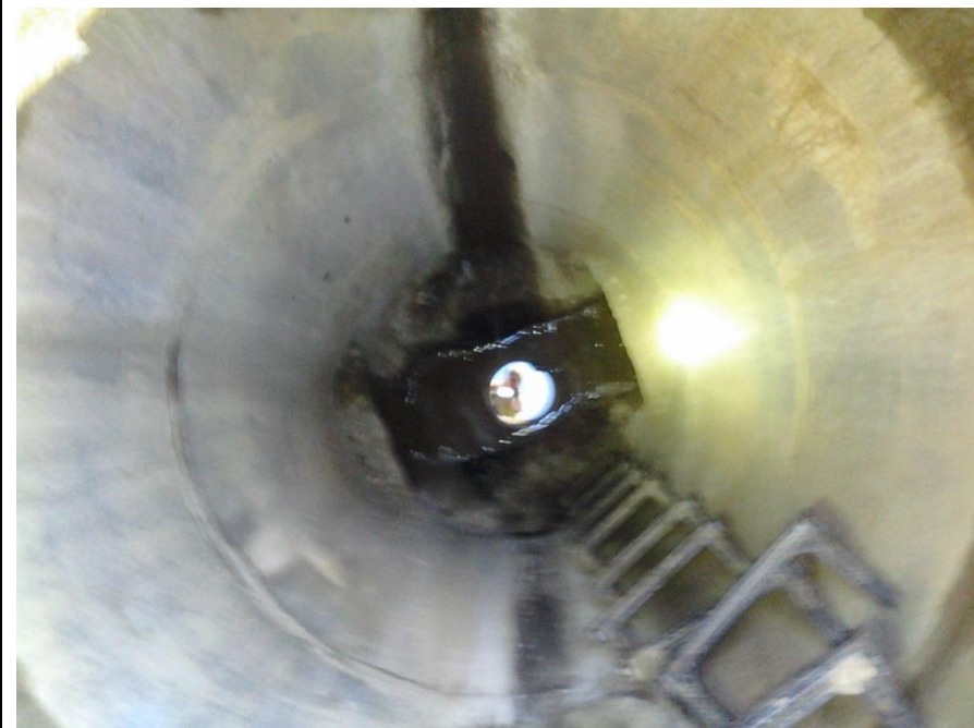
MH 6219 (119) @20963 Negaunee. Sampled flow in main channel from N. Staining on E. Wall. E&W Rd. Drain Inlets were dry
