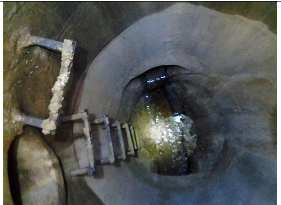
6192 (059) @ 21745 Seminole. W & E Road Drain Inlet were dry. Grey water, toilet paper, grease in flow from N. Sampled
