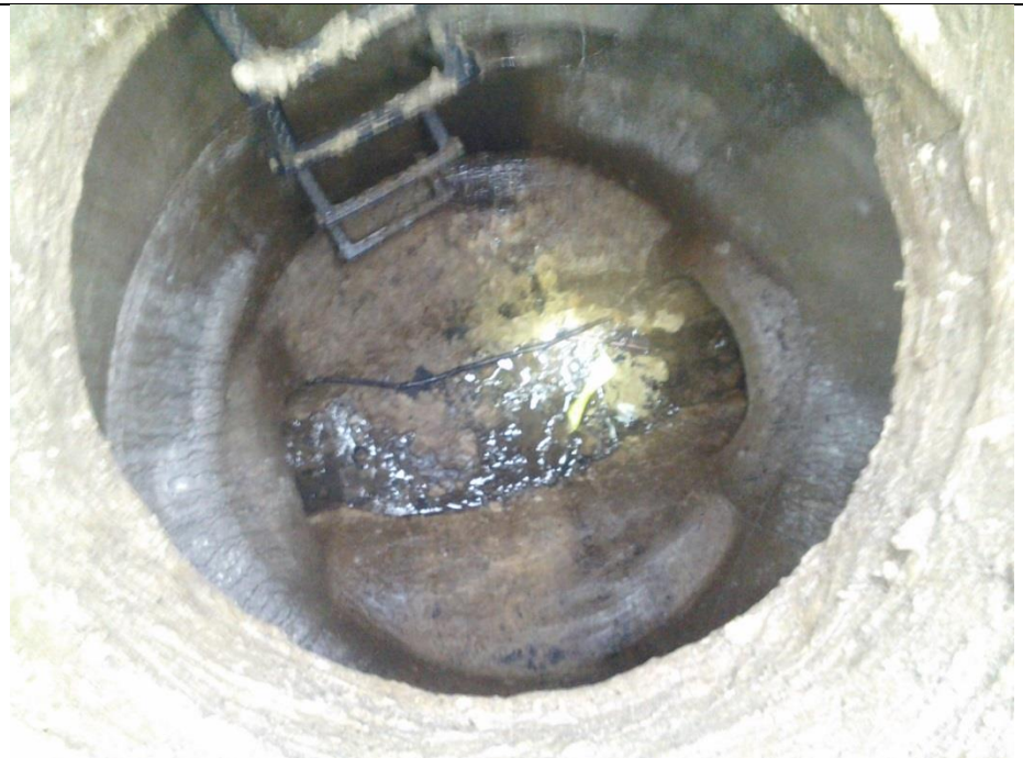
MH 6186 (018)@21596 Poinciana. Low flow in Main channel sampled. Possible grey water. E & W Rd. drain CB inlets were dry.
