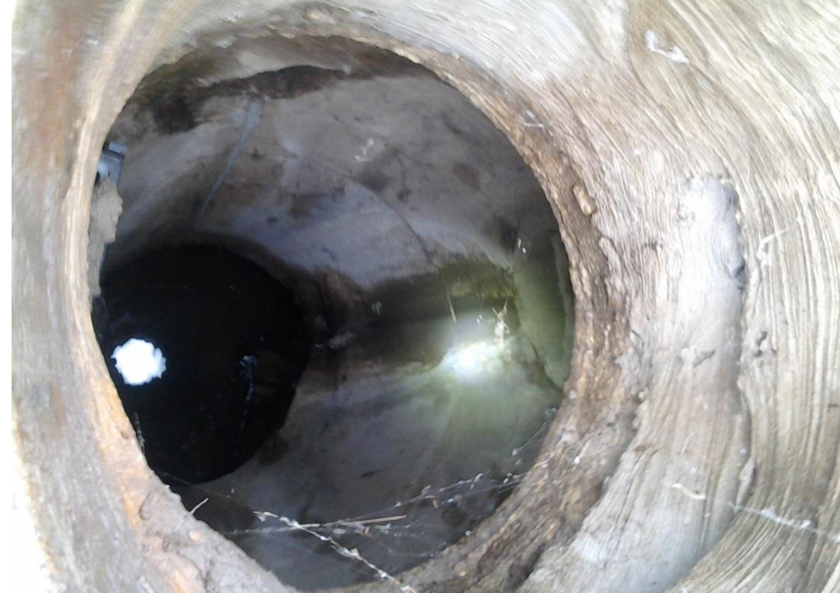
MH 6216 (101) Connects flow from west on Byron to East on Byron. Flow from N on Negaunee. Inlets from NE, NW & SW Road Drain Ditches. Trickle flow in NW Pipe. Sampled flow in channel
