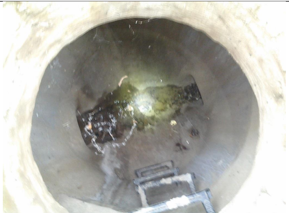
MH 6188 (030). Dry No Flow, N Inlet and E ,W Rd. drain CB Inlets were dry
