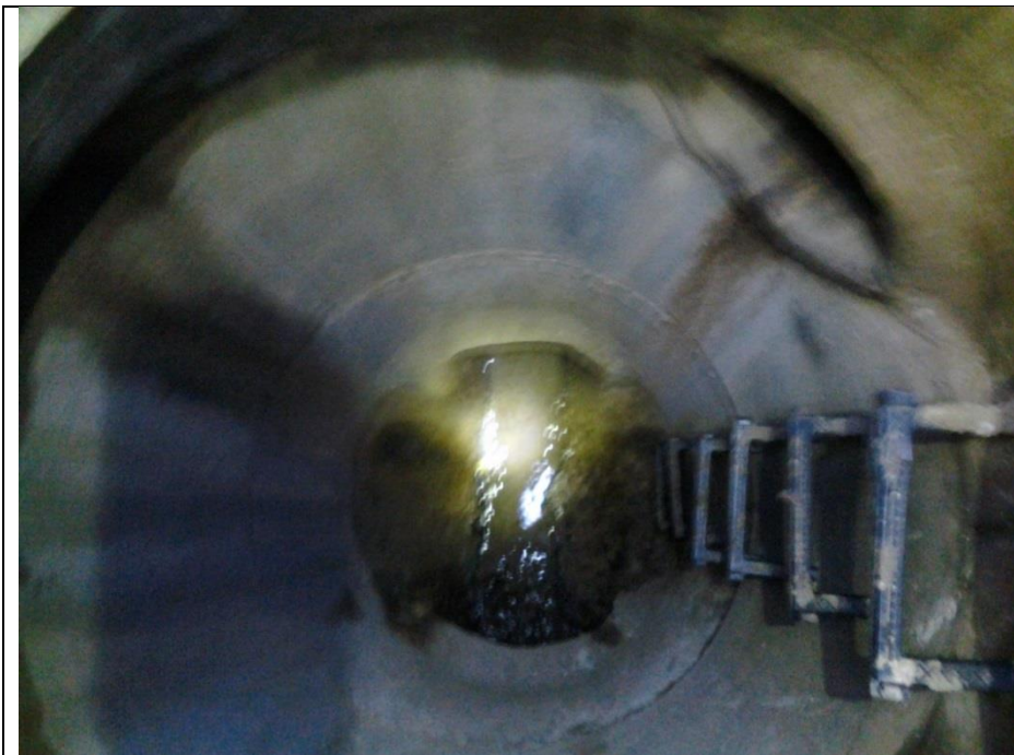
MH 6191 (053) @ Park on E. Seminole. NW & NE road inlets were dry. Flow from N. has grey water & possible toilet paper. Sampled
