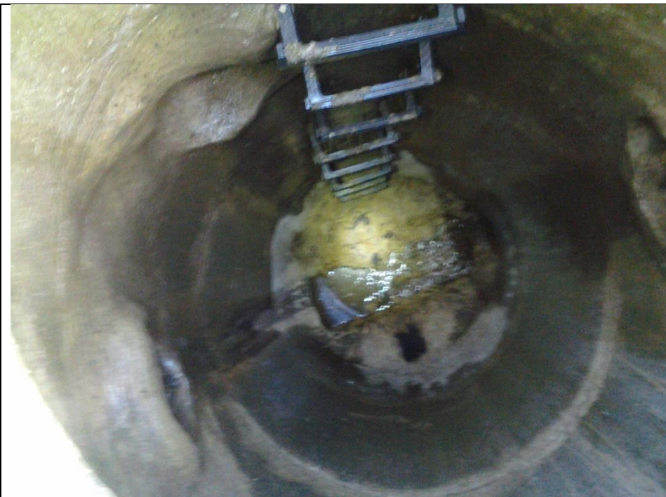
MH 6215 (091) Indian @ Shuiawassee Upper terminus. Dry No flow. Inlet form N, & SE, SW Road Drain CB Inlets were dry.
