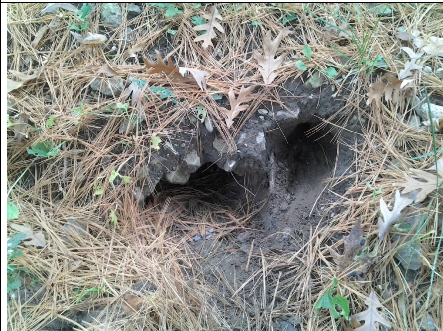
Ditch line N. of CB 13179 @ 21349 Poinciana. Possible Inlet to older drain system. Connection unknown.
