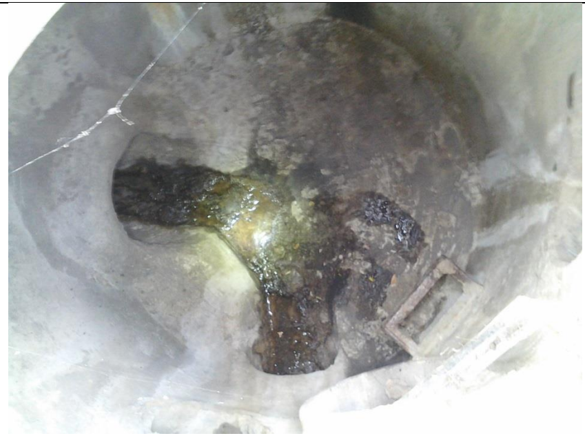
MH 6242 (298) @ Inkster Rd & Byron. Dry, No Flow. Connects N. to E on Byron. S. SE, N, W NE, NW Rd. CB Inlets were dry.
