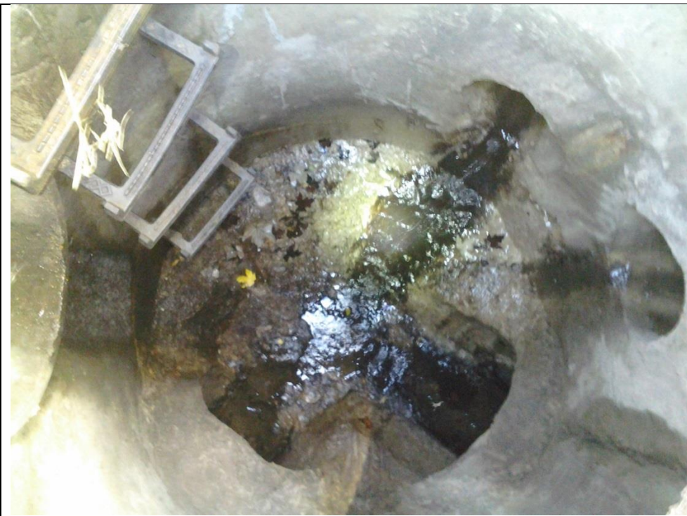
MH 6195 (081)@ Adeiline @ Inkster Rd. Upper Terminus with latreal connection to seminole St. E. Flow from N. connected local storm sampled. SW & NE Rd. Drain CB Inlets were dry.
