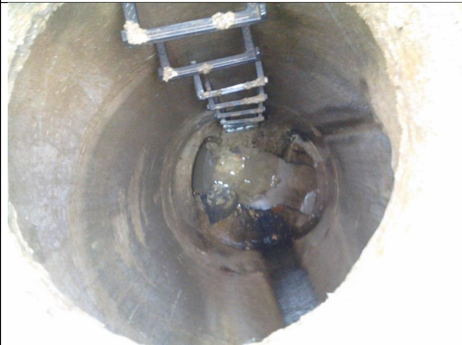
Ditch line N. of CB 13179 @ 21349 Poinciana. Possible Inlet to older drain system. Connection unknown.
