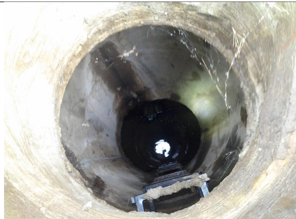
MH 6220 Emmett @ Negaunee (125) Sampled Flow from N. NE, NE, SE & SW Rd Drain inlets were Dry
