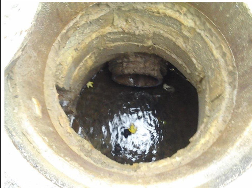
CB 13781 (232) Connected to MH 6233 (226). @27207 Shiawassee Inlets W&S. S Inlet has flow, possible sump connection
