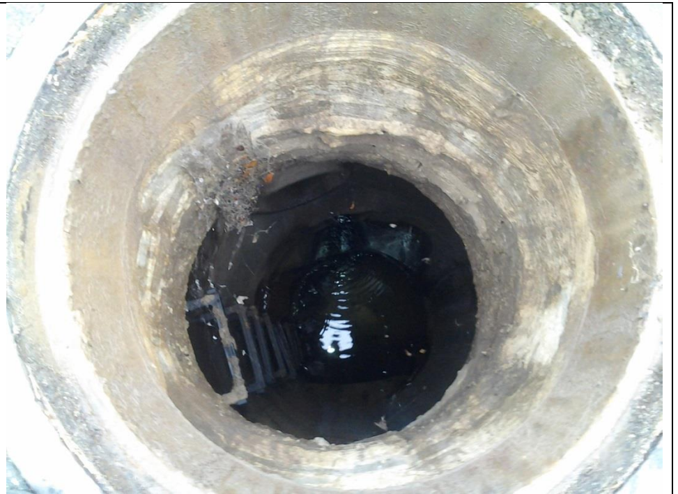
MH 6227(172) at Byron & Poinciana, connects flow from W on Byron to E on Byron. Flow from N. inlet on Poinciana. Inlets from NW, NE, SW & SE road drains were dry. Sampled main channel
