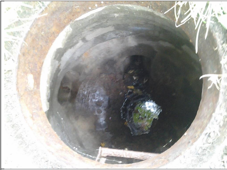
MH 6245 (309) Inkster Rd. at Emmett. N & S connections. Sampled Flow. Connection to Seminole St. Adjacent MH to W. not connected. NW, SW & NE Rd Drain CB Inlets were dry
