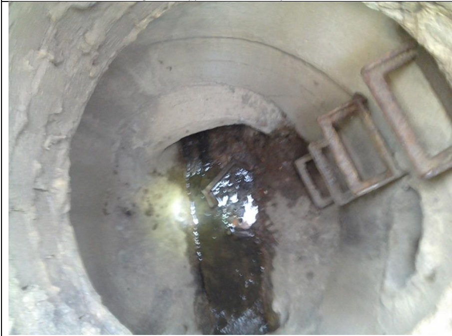
MH 6225 (165) N. Side of Shiawassee@ Negaunee. W & NE Rd. CB Inlets were Dry. Sampled flow from N. Possible sanitary debris
