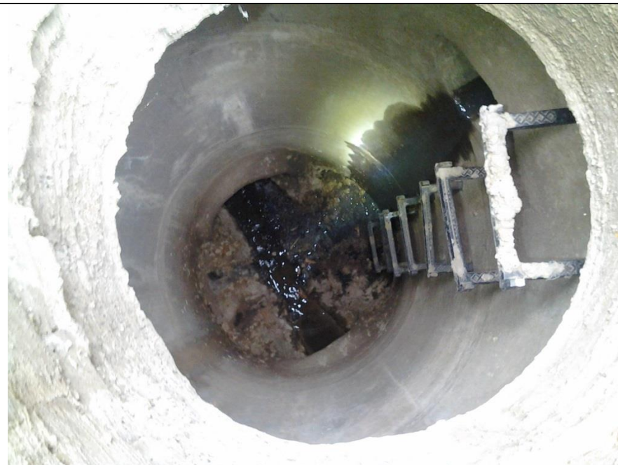
MH 6232 (220)@21349 Poinciana. W. Rd Drain CB w. flow & staining. Sampled flow in channel. Investigated CB 13179
