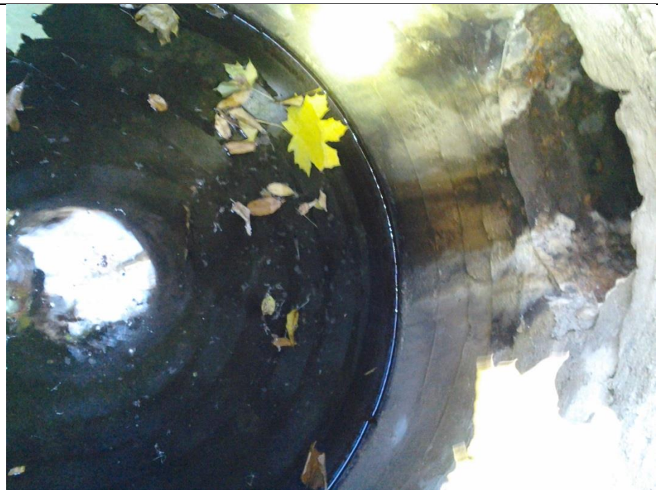
6223 B. CB 13779 connected to MH 6223 w inlet from N. from unknown drain. Sump sampled
