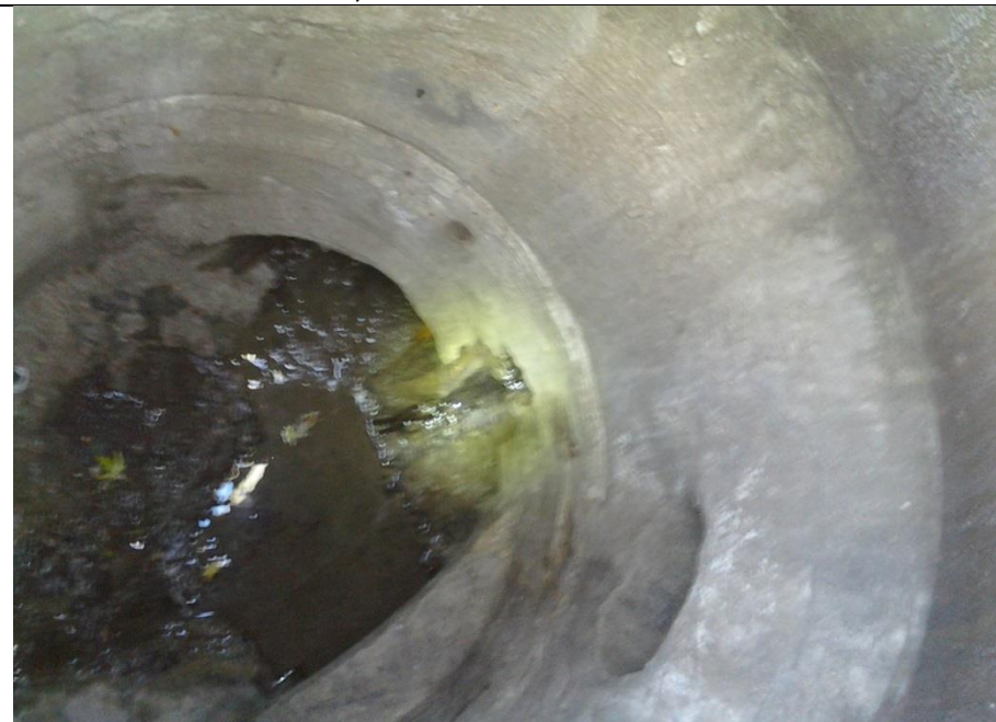
MH 6248 (321) Inkster Rd @ Sedalia. Flow From N. & S sampled. Lateral connection E. to Seminole St. unknown 6" connection with staining in NE corner of MH.
