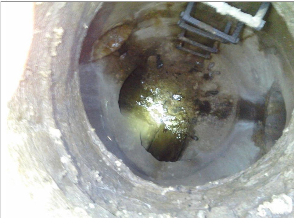
MH 6194 (071) Seminole & Adelein. Is N terminus for Seminole. NE, NW Road drain inlets were dry. Flow from W. on Adelein. Sampled.
