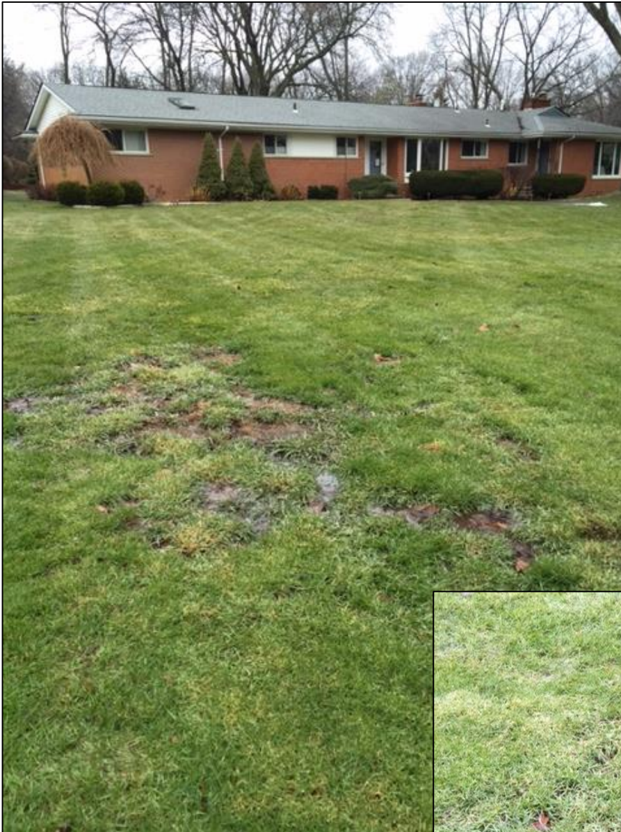
Figure 9: Photo of Failed Septic Field on Charing Cross
