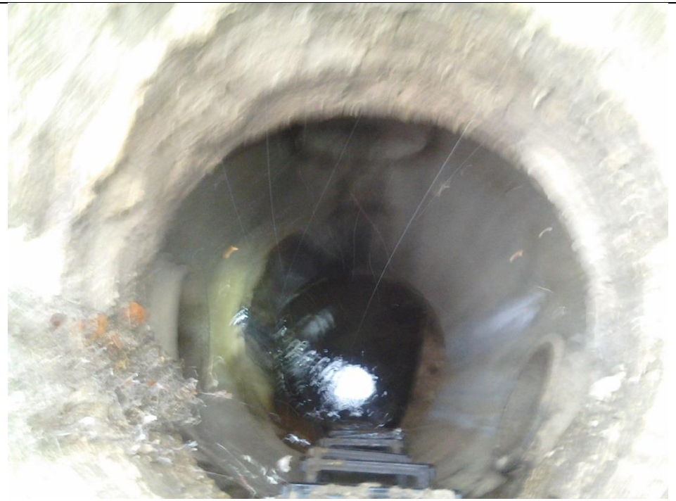
MH 6235 (237) at Byron and Seminole connect flow from W on Byron to E on Byron. Flow in N inlet on Seminole. Inlets form NE, NW, SE, SW road drains were dry. Sample main channel
