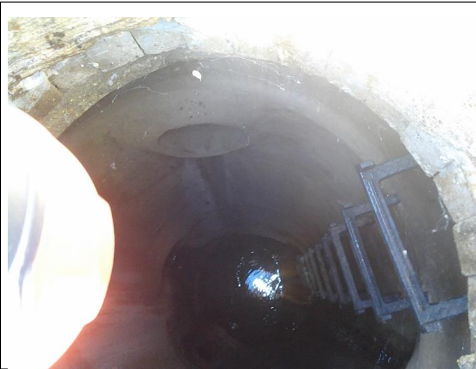
MH 6236 (253)@ 21048 Seminole connects flow N to S on Seminole. Inlets from SE, & SW road drains were dry. Sampled flow in main channel
