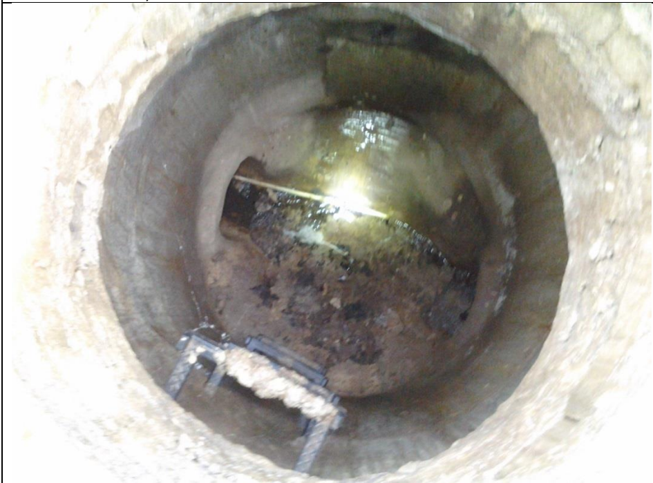
MH 6189 (036). @ Adelein & Poinciana.. Upper terminus MH for Poinciana. Rd. Dry no Flow Drain inlets were dry.
