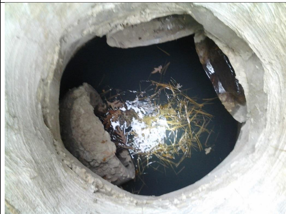
CB 13179 Connected to MH 6232 (220). @ 21349 Poinciana. Grey water in sump. Sampled. Inlets from W & S
