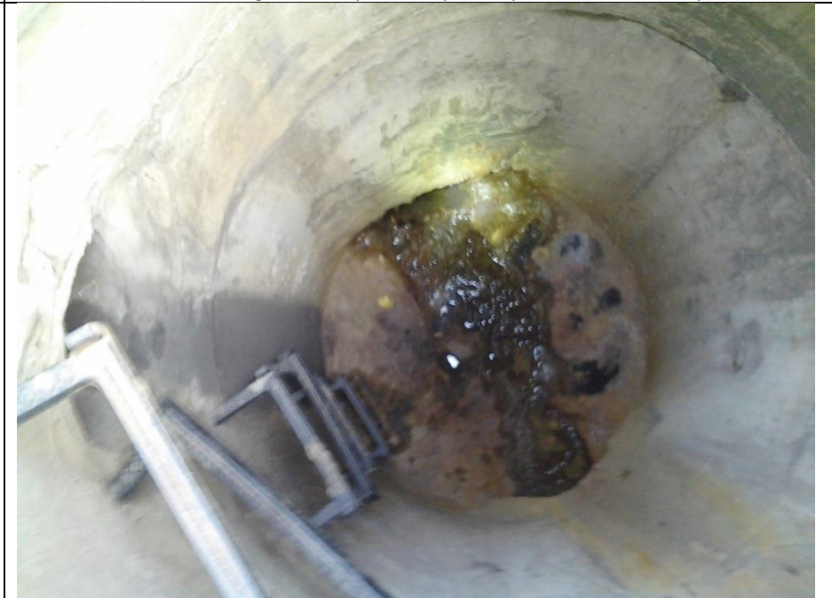
MH 6224 (157) S. Side of Shiawassee @Negaunee. Sampled. Flow from N. W & SE Rd CB Inlets were dry. Possible toilet paper up in pipe. Sampled
