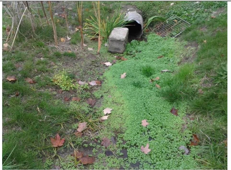
Flow from driveway culvert to ditch line S to inlet 13746 (111). Could hear gurgling sound coming from up in culvert. Flow sampled. Probably a connected sump pump. Sampled flow.
