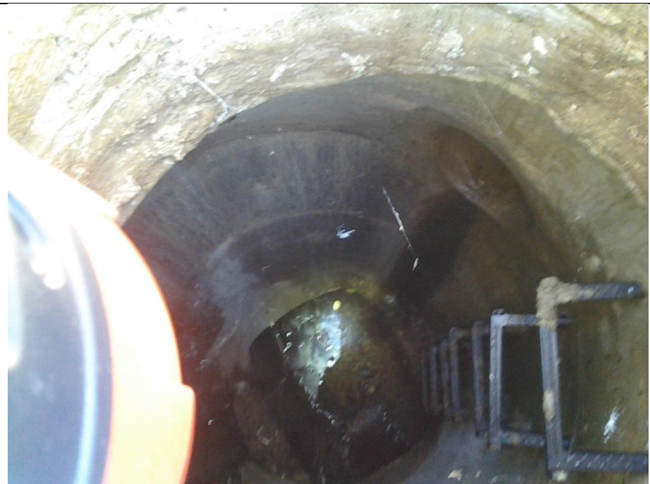
MH 6240 (269) @ 21351 Seminole, SE, SW road drain inlets were dry, Toilet paper, grease ,sanitary, in flow from N. Sampled
