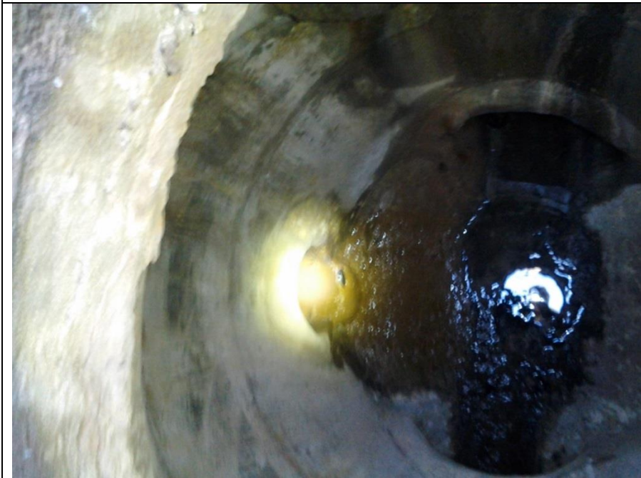
Tap with flow from W. tied into MH 6193 (065). Pipe runs under driveway for 21823 Seminole. May be an illicit connection
