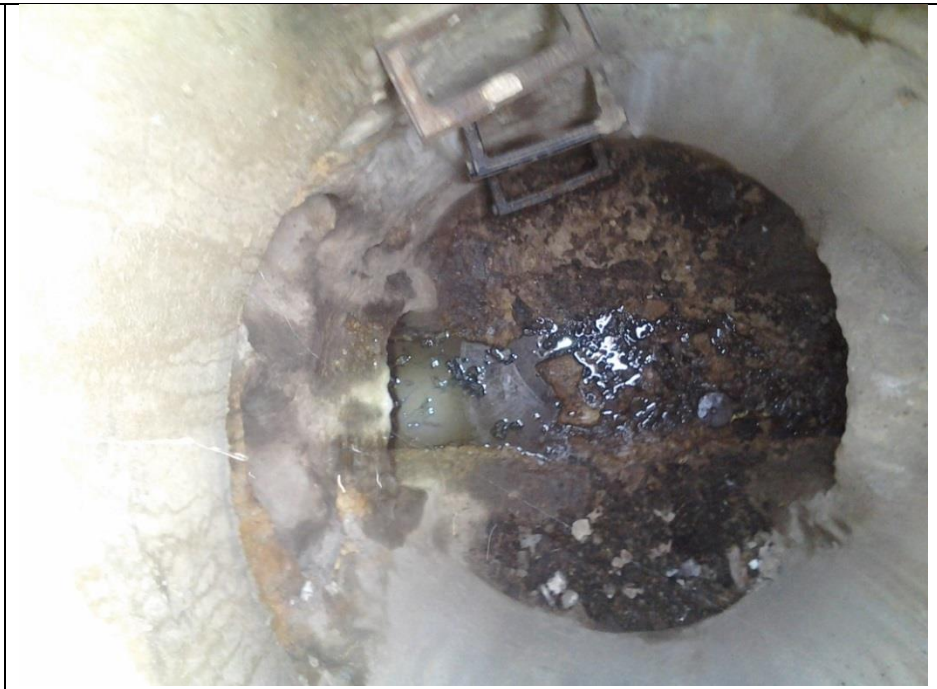
MH 6183 (001) @21545 Negaunee,. Dry MH. Grey water pooled in outlet. Sampled
