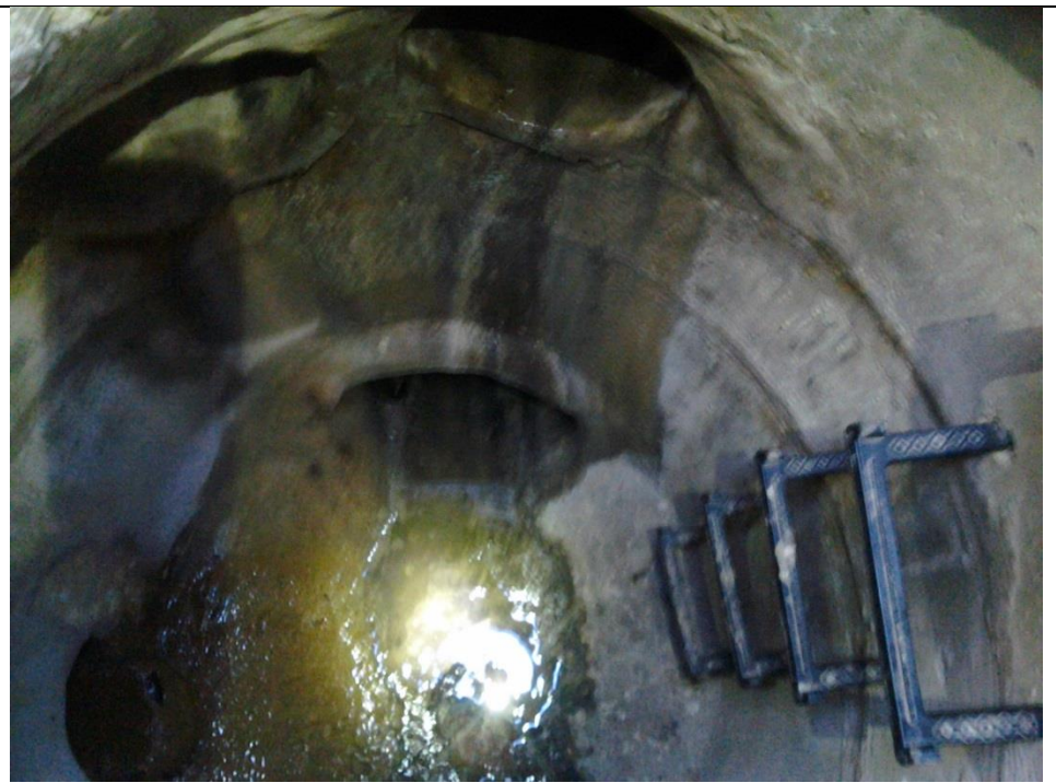
MH 6193 (065) @ 21847 Seminole. NW, NE road drain inlets were dry. Flow from N has grey water. Inlet from W has flow w possible sanitary pipe is under driveway at 21823 Seminole.
