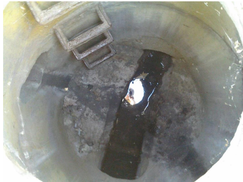
MH 6201 (107) @ Shiawassee & Inkster Rd.SE Corner. Flow in Main Chanel From N. Sampled. SE & W Rd. Drain CB inlets were dry.
