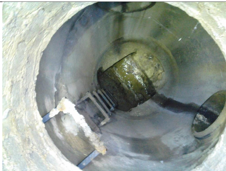
6223 B. CB 13779 connected to MH 6223 w inlet from N. from unknown drain. Sump sampled
