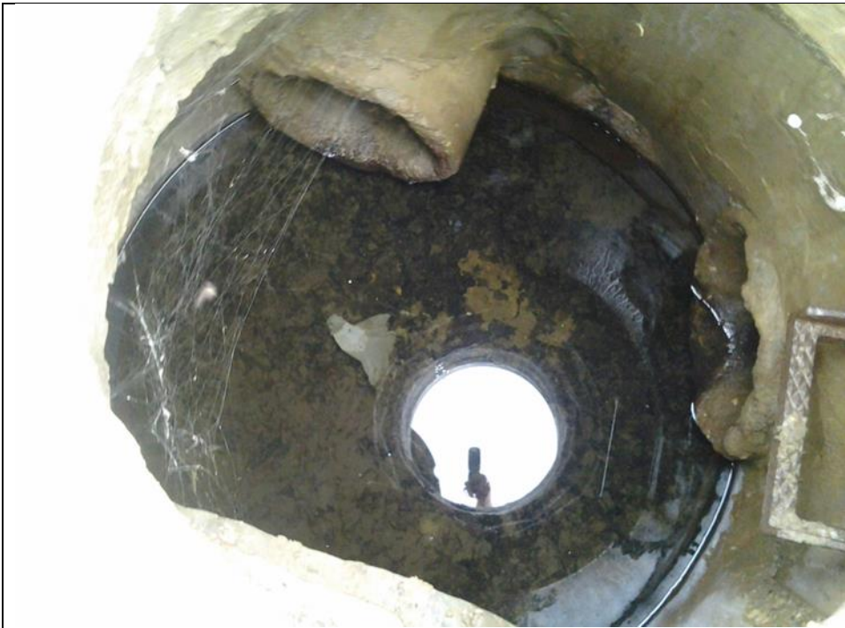
CB 131467 (111) on E side of Negaunee, has flow from drainage ditch culvert in front of 20912 Negaunee. Sampled CB
