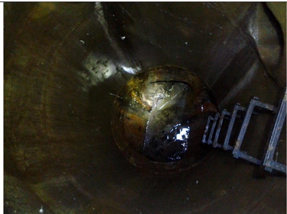
MH 6190 (045) Shiawassee @ Seminole. MW,NE,SW,SE Inlets for road drain ditches were dry. Additional E&W inlets for Shiawassee Rd. (not in GIS) w staining. Flow from N .has toilet paper
